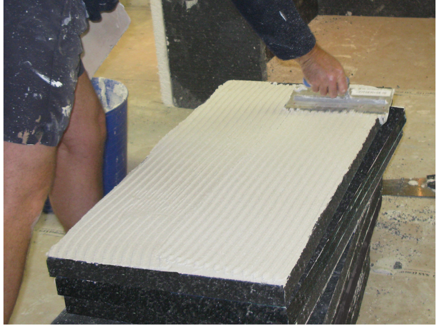
Figure 3 - Adhesive Application
